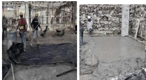
Figure 34. Casting of the floor plate
