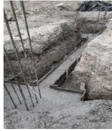
Figure 16. Casting of foundation beams
