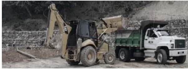
Figure 4. Mechanical site clearance.
