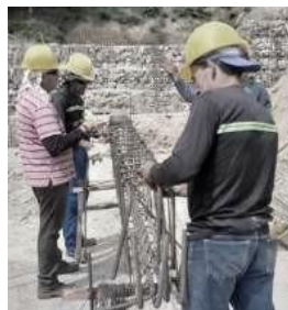
Figure 15. Steel reinforcement of the foundation beams
