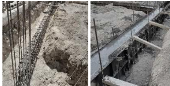
Figure 24. Assembly and casting of the tie beams
