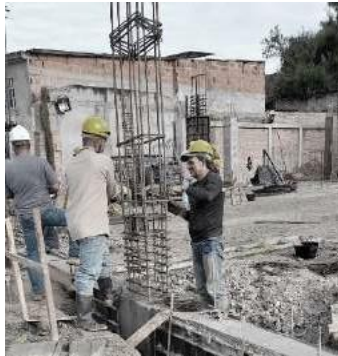
Figure 27. Steel reinforcement of columns
