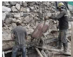
Figure 25. Tie beam casting with 3000 PSI concrete
