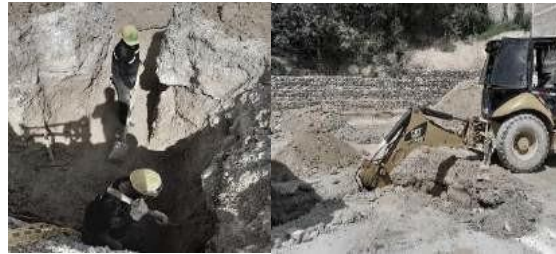
Figure 11. Manual and mechanical excavation of foundation beams
