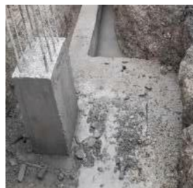
Figure 19. Cast pedestal.
