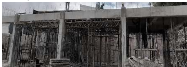
Figure 31. Casting of overhead beams
