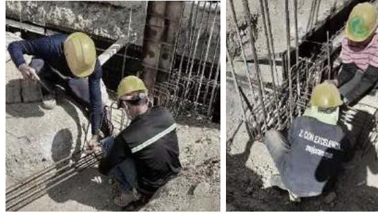
Figure 23. Assembly of the tie beams
