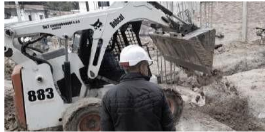
Figure 20. Mechanical backfilling of the excavation with common material
