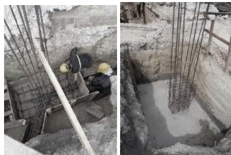
Figure 14. Shoe casting
