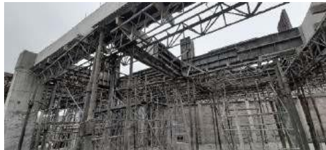
Figure 30. Assembly and formwork of the overhead beams
