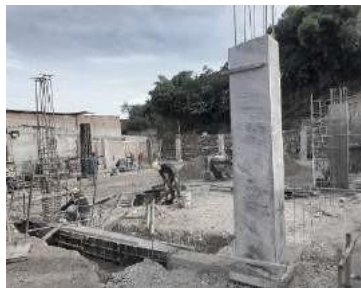
Figure 28. Column casting
