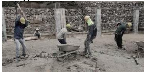
Figure 33. Levelling of the terrain
