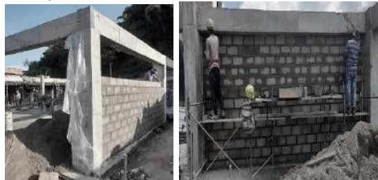
Figure 36. Masonry work
