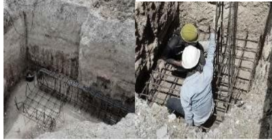
Figure 13. Steel reinforcement of the footings.
