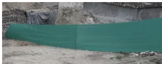
Figure 6. Temporary enclosure of the construction site in green tarpaulin.
