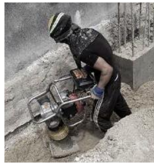
Figure 21. Compaction of the backfill with a kangaroo rammer.
