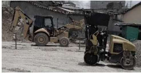
Figure 7. Excavation and compaction
