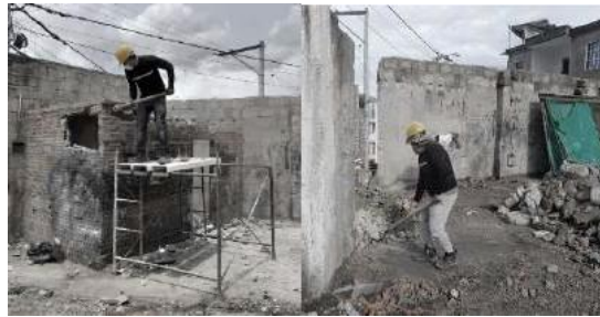
Figure 2. Manual demolition of existing buildingsite.
