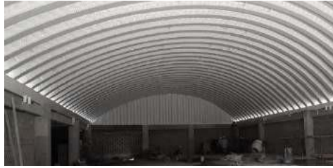
Figure 37. Installation of self-supporting roof
