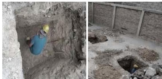
Figure 9. Excavation of footings at a depth of 2 metres.
