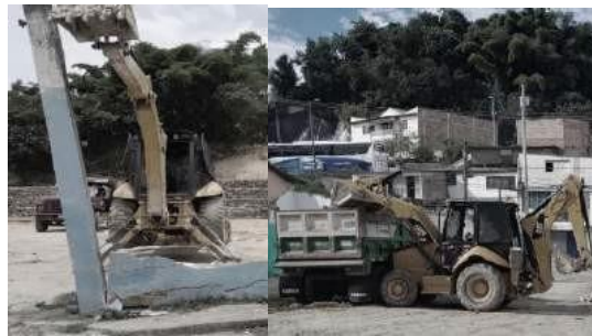
Figure 3. Mechanical demolition of existing works
