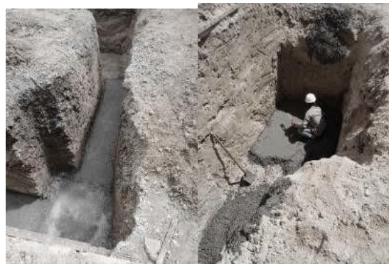
Figure 12. Cleaning screeds
