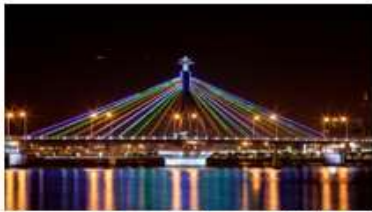
Figure 3: Han River Bridge
