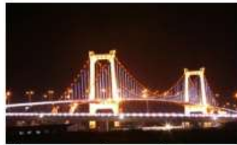
Figure 4: Thuan Phuoc Bridge
